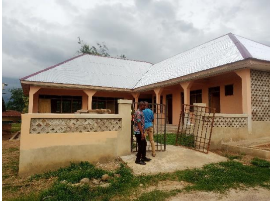
Two Unit Classroom block with auxiliary facilities and furniture
